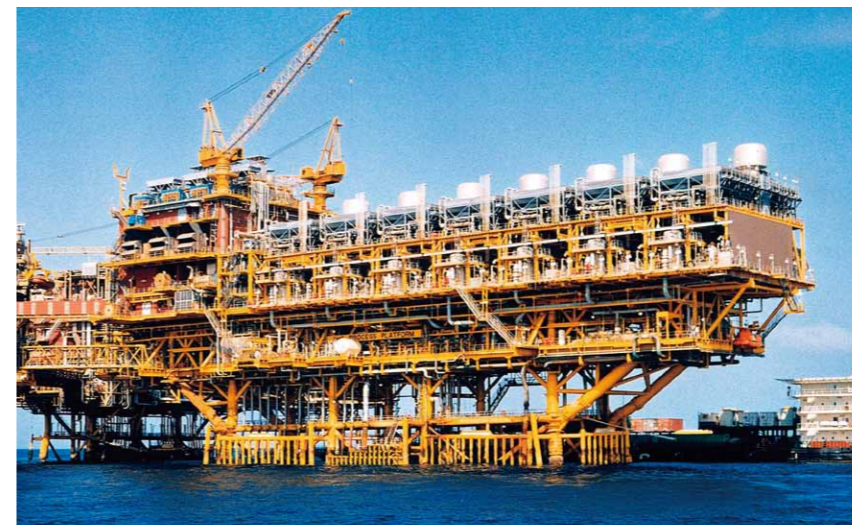
Gas compression module for offshore platform (India)
