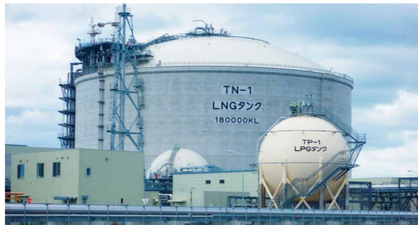
Full containment tank
