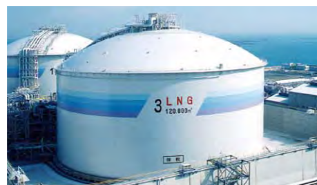
Single containment tank
