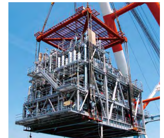
Gas compression module for offshore platform (Shipping out from Kobe Works)
