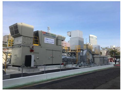
Demonstration plant of hydrogen-fueled gas turbine cogeneration system
