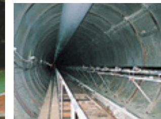
Ring beam supports
