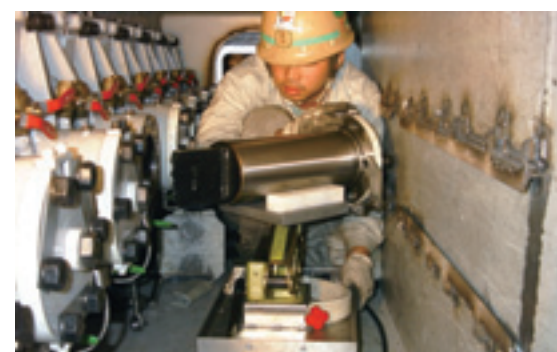
During cutter change from inside
