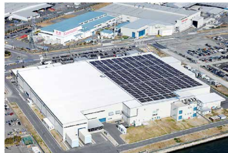
Figure 9: Nagoya Works 1: 750-kW power generation facility
