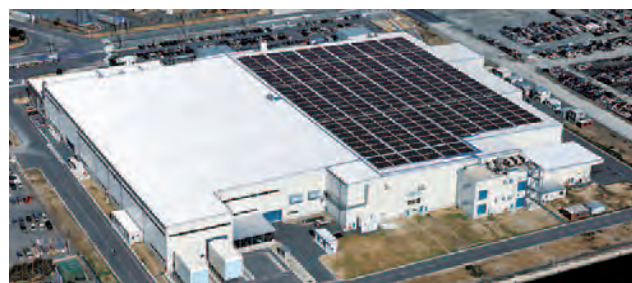
Nagoya Works 1: 750-kW power generation facility
