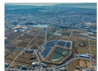
Iwaoka Photovoltaic Power Generation Station
