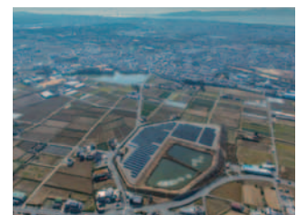
Iwaoka Photovoltaic Power Generation Station
