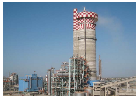
Urea manufacturing facility
