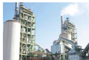
Cement plant waste heat recovery power generation
