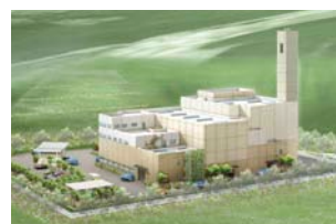
Waste Incineration Plant
