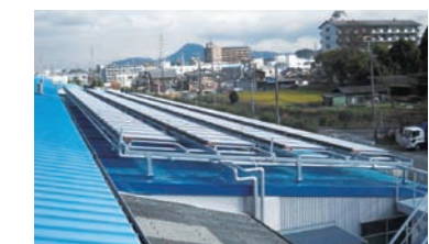
Solar cooling system—an integrated system using solar heat and an absorption-style chiller to provide highly efficient heating and cooling for factories and large commercial buildings
