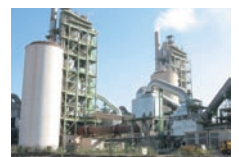
WHRPG in cement plant in Pakistan
