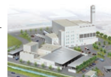
Combined waste incineration/biogas generation complex
