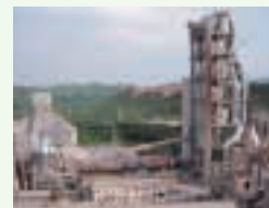
WHRPG in cement plant
