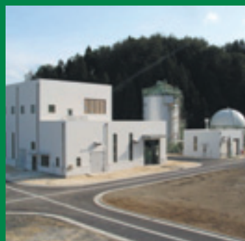
Delivered to Suzu city, Ishikawa prefecture
