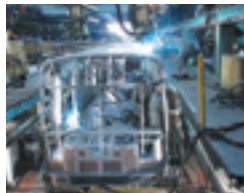
Rolling Stock Company Hyogo Works
