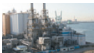
■ Energy/Environmental Preservation Facilities
