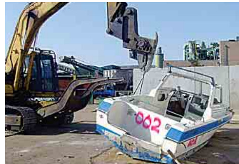
Dismantling of FRP Boats
