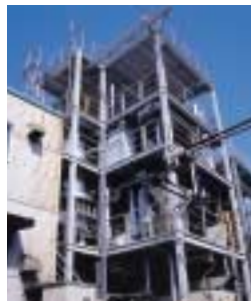
Test plant during tests of gasification reaction characteristics
