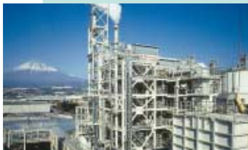
RPF burning waste power generation plant The capacity is one of the largest in Japan, burning 330 t/day of paper sludge and 50 t/day of RPF.
