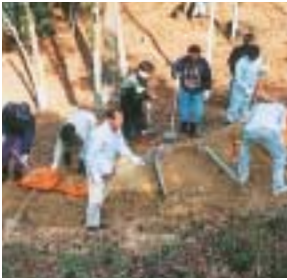
Maintenance of Yashiro-no-mori Park in Hyogo Prefecture
