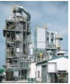
Internal circulation fluidized bed-type incineration system
