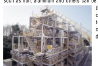
this way, effective resource recovery can be performed. High temperature melting at a cyclone furnace enables to control dioxin formation.
