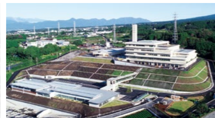
Municipal waste incineration plant
