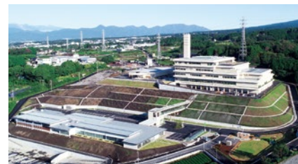
Municipal waste incineration plant
