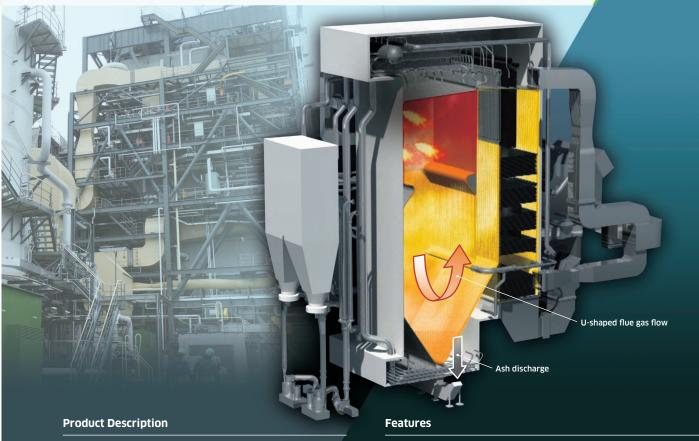
A boiler that can achieve mono-firing of combustion-resistant petroleum residues, such as petroleum coke and asphalt pitch, with no need for auxiliary fuel (electricity output: 36,000 kWe) The U-shaped flue gas flow at the furnace bottom encourages ash to separate from the flue gas
