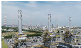
KG-18-T 100 MW-class combined cycle power plant
