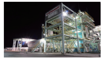
Hydrogen liquefier used for demonstration operation
