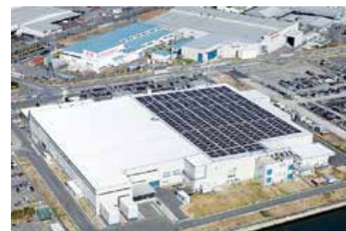
Figure 13: Nagoya Works 1: 750-kW power generation facility
