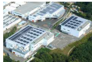
Figure 14: Nishi-Kobe Works: 927-kW power generation facility (of which 422 kW are sold via FIT)
