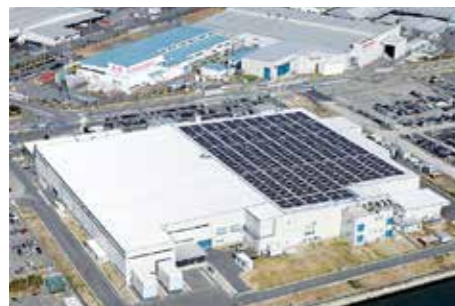
Figure 13: Nagoya Works 1: 750-kW power generation facility
