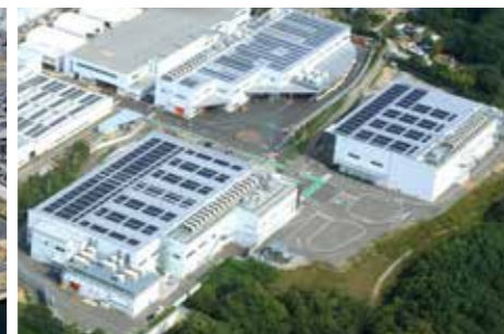
Figure 14: Nishi-Kobe Works: 927-kW power generation facility (of which 422 kW are sold via FIT)
