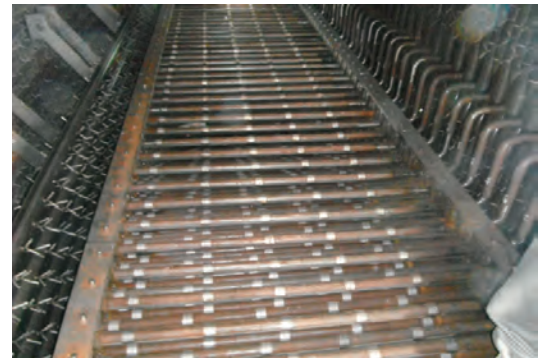
Fig. 3 Embedded tubes
