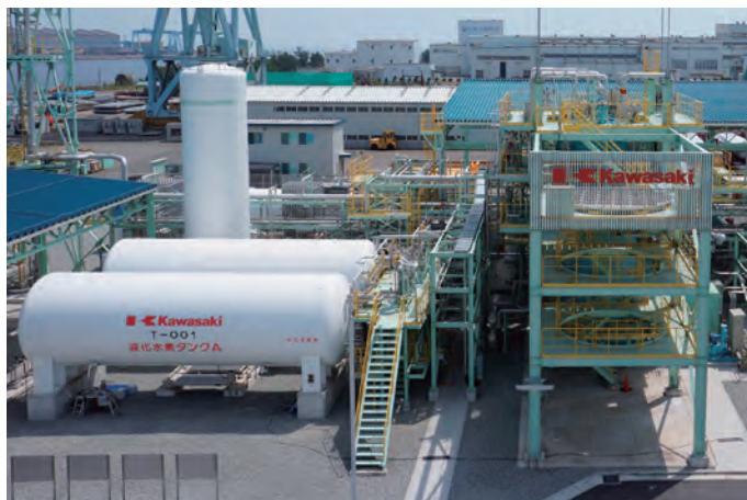
Fig.3 Japan's first-large scale hydrogen liquefier
