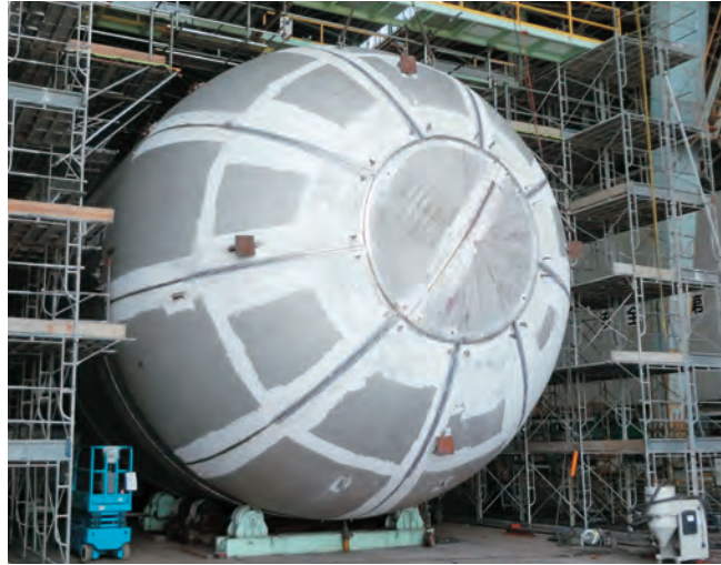
Fig.5 Trial manufacture of aboveground LH 2 tank
