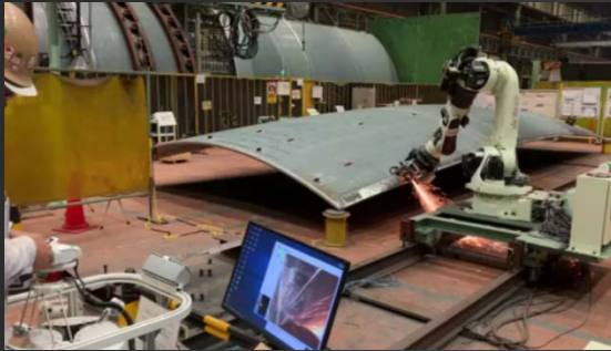
Grinding work (Development of a remote control system using 5G)
