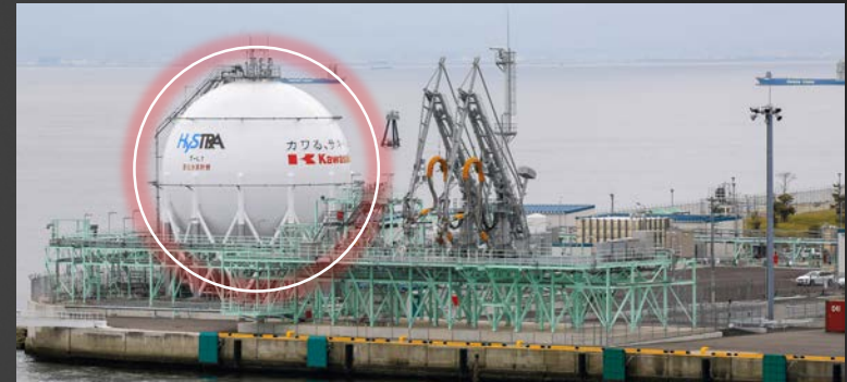
Japan's largest liquefied hydrogen storage tank
