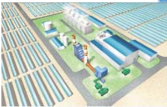
Integrated Solar Combined Cycle power generation system ■ Solar Heat + Gas Turbines, etc. ■ Deployment in Middle East market
