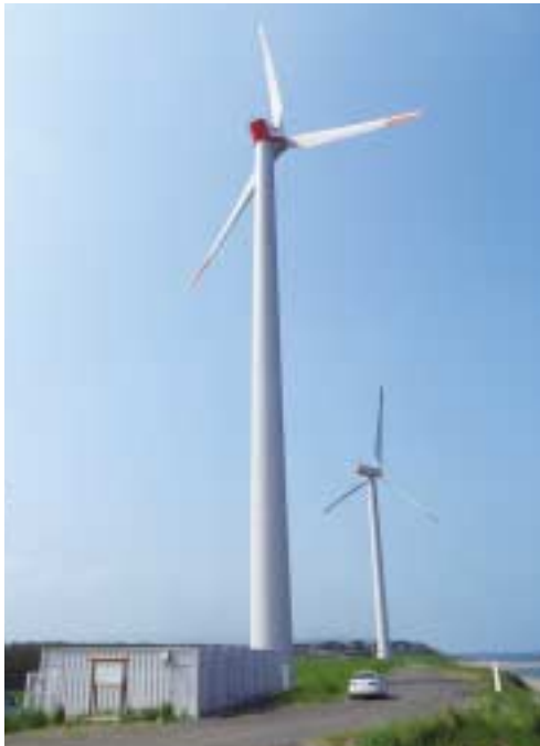
Wind power generator at Win Power Nishime Wind Farm.
