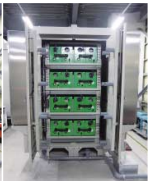
The GIGACELL system used in the microgrid of the Shimizu Corporation Technical Research Center consists of a string of 16 modules.
