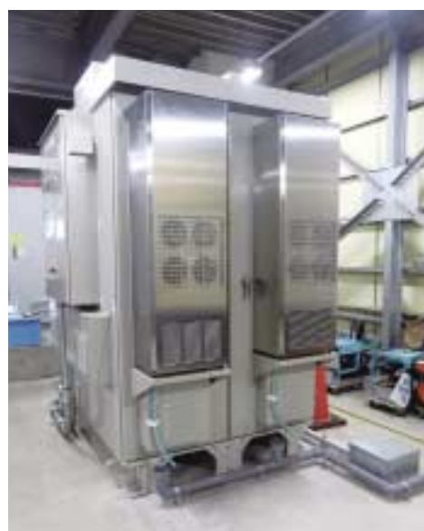
The GIGACELL system used in the microgrid of the Shimizu Corporation Technical Research Center consists of a string of 16 modules.
