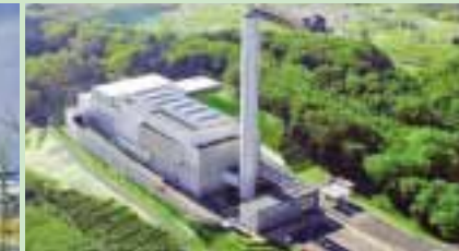
Hirakata Tobu Waste Incineration Plant Daily incineration capacity: 240t (120t x 2 furnaces) Power-generating capacity: 4,500 kW Completed: December 2008
