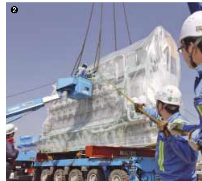
Construction of the power plant proceeds (Photo 1) while Kawasaki Green Gas Engines are brought in (Photos 2 & 3) to the Sodegaura Green Power construction site. All 14 engines at the power plant are slated to begin operation by mid-August of this year. It will have taken just one year to get a 110 MW power plant operating, thanks to the short lead time of the Green Gas Engine.
