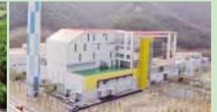
Gumi City MSWIP*, South Korea Daily incineration capacity: 200t (100t x 2 furnaces) Power-generating capacity: 2,940 kW Completed: December 2010
