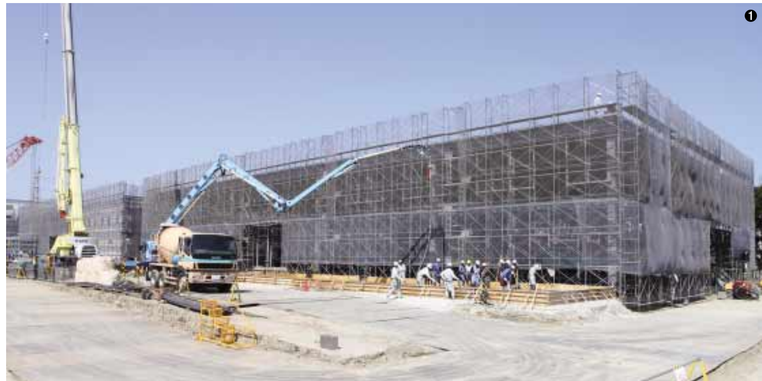
Construction of the power plant proceeds (Photo 1) while Kawasaki Green Gas Engines are brought in (Photos 2 & 3) to the Sodegaura Green Power construction site. All 14 engines at the power plant are slated to begin operation by mid-August of this year. It will have taken just one year to get a 110 MW power plant operating, thanks to the short lead time of the Green Gas Engine.
