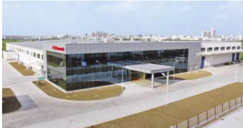
Kawasaki's new plant began full-scale operations on Nov. 1, 2011. It can produce 60,000 hydraulic pumps and 50,000 hydraulic motors a year, twice the capacity of the old plant.
