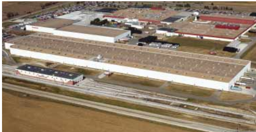
The KMM Lincoln plant, the newest and largest rail car facility in the U.S. and the only one designed for integrated mass production of subway, commuter and high-speed rail cars.
