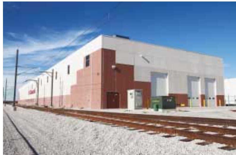
The Lincoln plant now has functional and operational test facilities with 600 m of test track.
