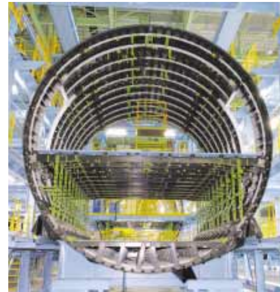
The inside of the forward fuselage still looks quite bare. The top half will be the passenger cabin while the bottom half will be used as cargo space.
