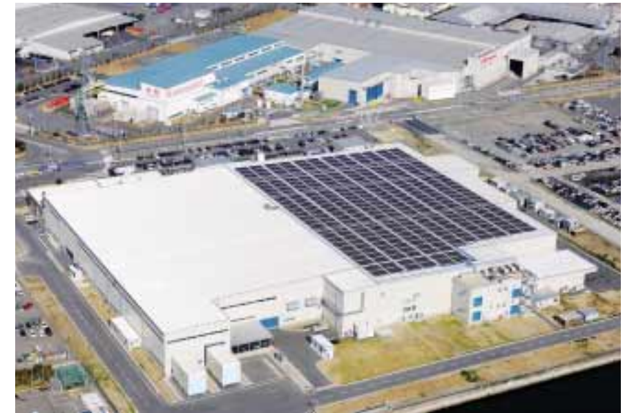
Overview of the Nagoya Works 1. The gray-roofed building (upper right) is the 787 North Plant. In the foreground is the 787 South Plant, with a rooftop solar-power system that generates 750 kW and can supply approximately 5% of the electricity consumed at the Nagoya Works 1.
