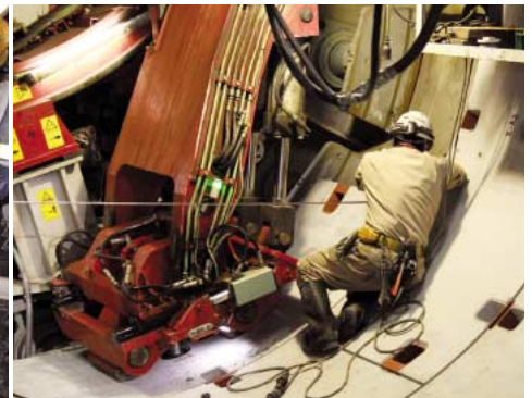
The unique cross-section demands precision accuracy when laying segment blocks.
