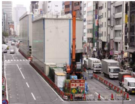
Street-level noise enclosure. The tunnel is being built toward the background.
