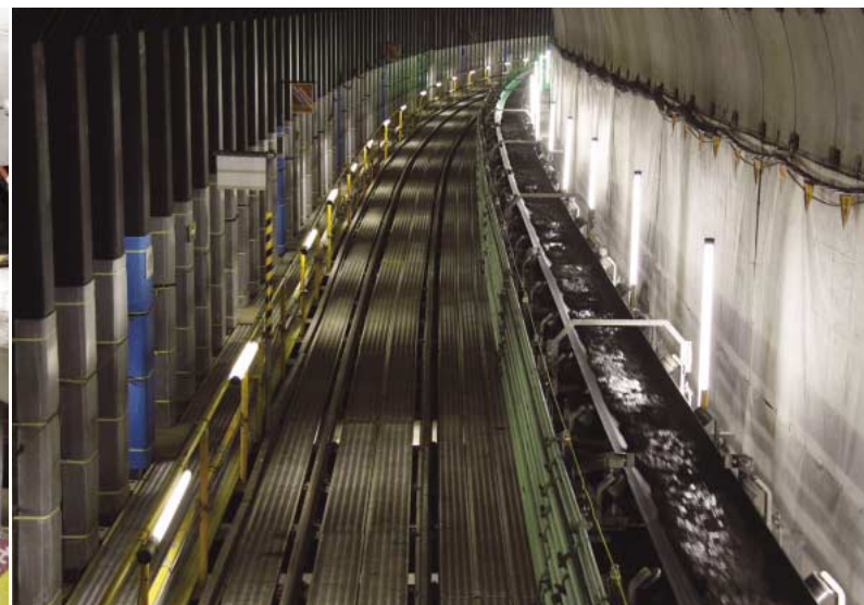
A completed section of tunnel. The other (identical) half of the tunnel lies to the left of the supporting columns.
