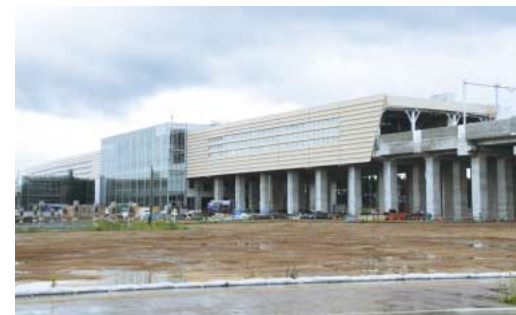
Shin Aomori Station, currently under construction.
