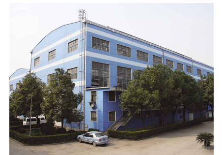
WKM factory buildings. Pictured in front is the assembly/testing shop.
