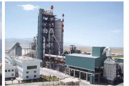
Kelete Cement Plant (clinker output: 3,000 t/day), Turkmenistan, 2005
