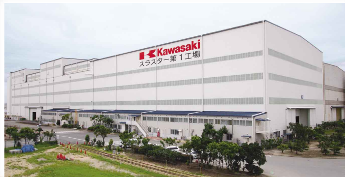
Exterior of Side Thruster Plant No. 1 (total floor area: approximately 10,000 m 2 ), Kawasaki's thriving production base at its new Harima Works home.
