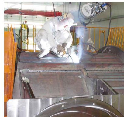
▶ The tube's sides are welded together with reinforcing ribs.
