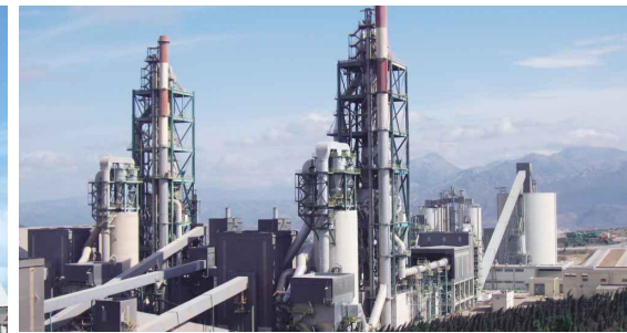
Lafarge Cement Plants (combined clinker output: 4,600 t/day), Morocco, Plant 1 (left) 2004 and Plant 2 (right) 2009
