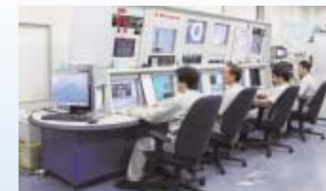
Test facility control room. A four-person test crew working in two shifts runs engine tests between 7:00 a.m. to 9:00 p.m.
