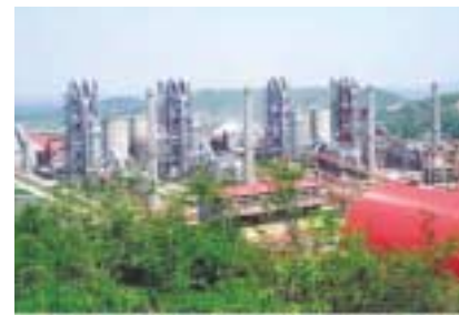
Wuhu Conch Cement Plant.
