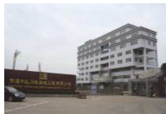
NACKS office building.
