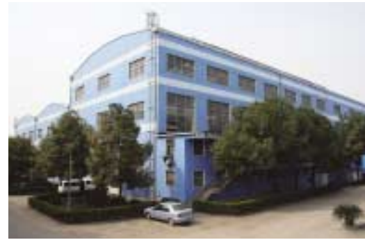
WKM factory buildings. Pictured in front is the assembly/testing shop.
