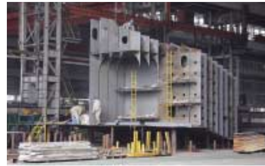
Large block units are assembled in the assembly shop.
