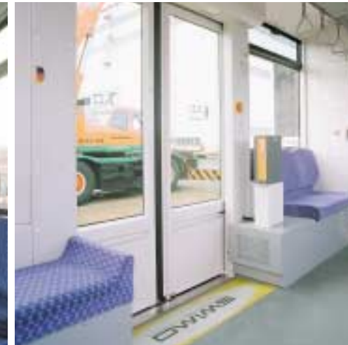
Sliding plug doors are located in the center of a passenger cabin. Batteries are installed under the seats.
