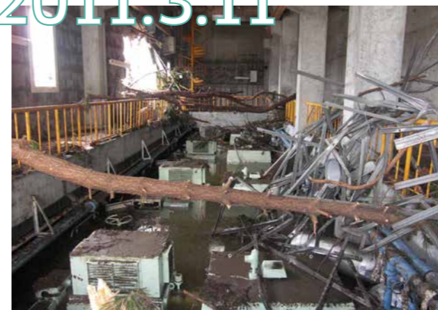
(Left) On March 11, 2011, the MGWTP was severely damaged by a giant earthquake and a tsunami which swept away much of its equipment and facilities. After the tsunami subsided, the blower bodies and pipes were found submerged in seawater inside the blower/pump station building, while floating debris had damaged various pieces of equipment. (Right) A temporary blower/pump station building was constructed in October 2012, housing two of 11 submerged blowers which had been disassembled, repaired, and reassembled, as well as a prototype of the MAG Turbo M35.
