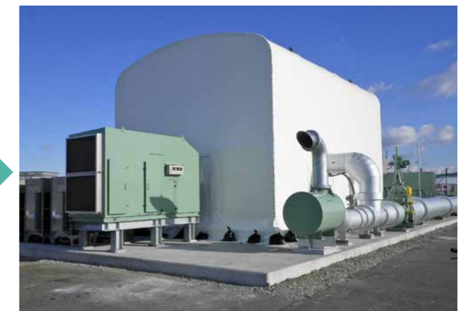
(Left) On March 11, 2011, the MGWTP was severely damaged by a giant earthquake and a tsunami which swept away much of its equipment and facilities. After the tsunami subsided, the blower bodies and pipes were found submerged in seawater inside the blower/pump station building, while floating debris had damaged various pieces of equipment. (Right) A temporary blower/pump station building was constructed in October 2012, housing two of 11 submerged blowers which had been disassembled, repaired, and reassembled, as well as a prototype of the MAG Turbo M35.
