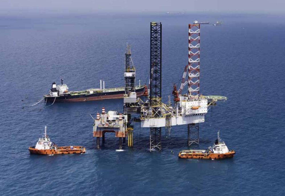
Under a platform standing in the ocean, multiple oil wells are scattered around.
