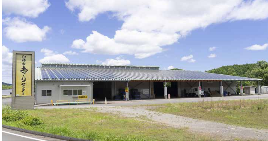
The Usuki Soil Manufacturing Center, located in the Notsu District, Usuki City, is a central facility for achieving an eco-system through organic farming.
